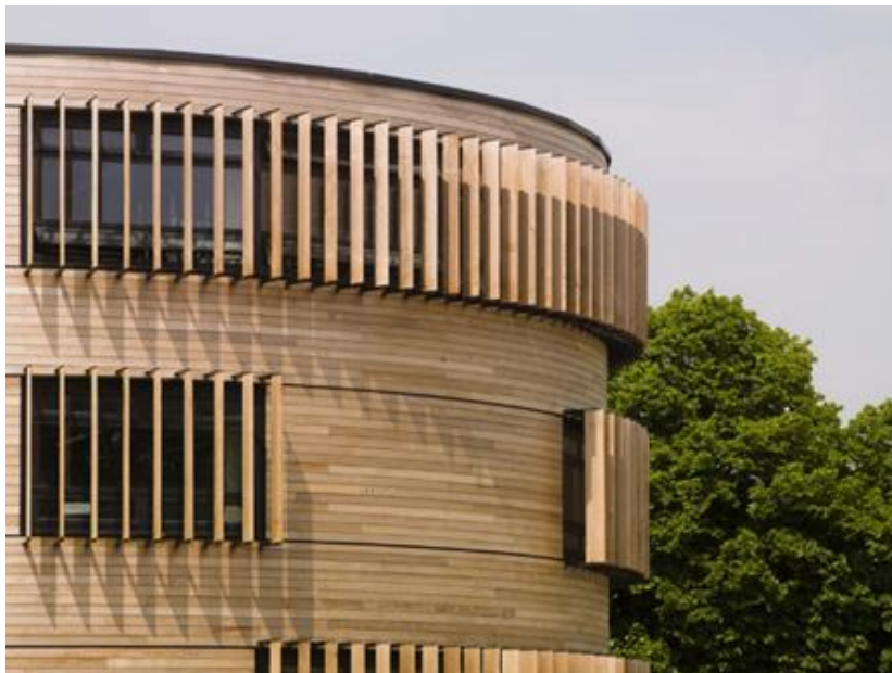
Fig 3: vertical wooden fins attached to curved building face Langley academy (Patrick Hislop & Philip O'Leary).
