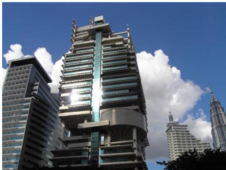
Fig 7: menara prudential Kuala Lumpur one of new high rise buildings which attempt to implement sun shading devices as eco-friendly design approach
