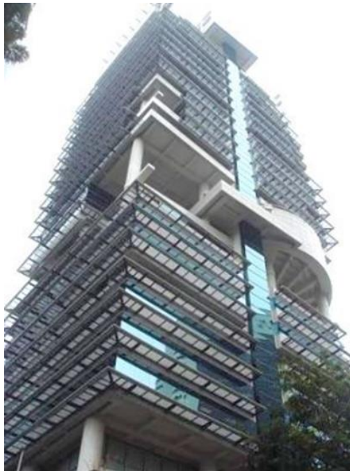
Fig 8: shading devices extruding out from the building diffusing sunlight before penetrating the building. (Google image)
